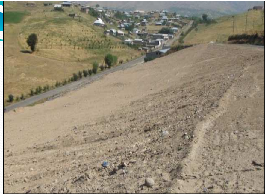
Photo 2 Sprinkle of body dump by layer of soil
